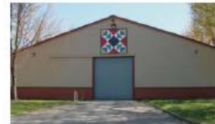
6 SERPILIO HALL Plumas Sierra County Fairgrounds 204 Fairgrounds Road BQ Pattern: Wild Goose Date of barn construction - 1961
