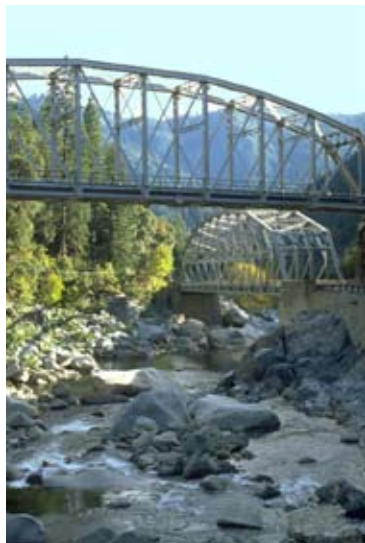
The Tobin Twin Bridges -- where railroad crosses over highway -- are among attractions along the Feather River National Scenic Byway.
