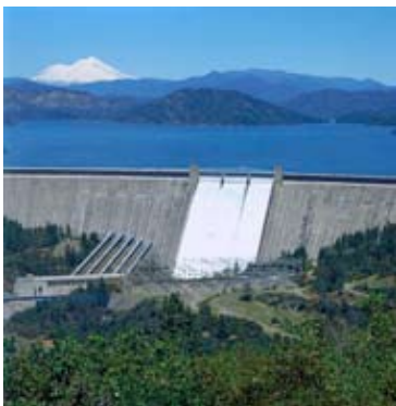
The three Shastas: Shasta Dam, Shasta Lake and Mount Shasta
