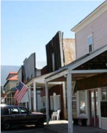
Greenville's Historic Main Street
